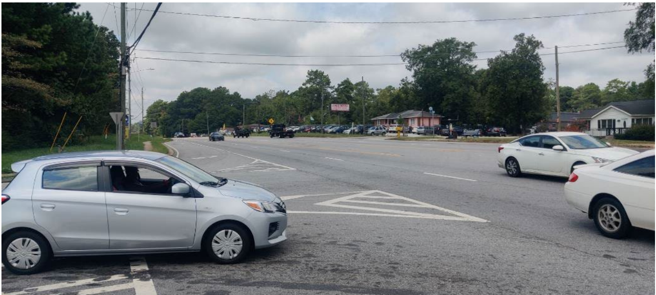
Figure 7-5: Lack of crosswalk at Park Central Rd & Covington Highway Intersection
